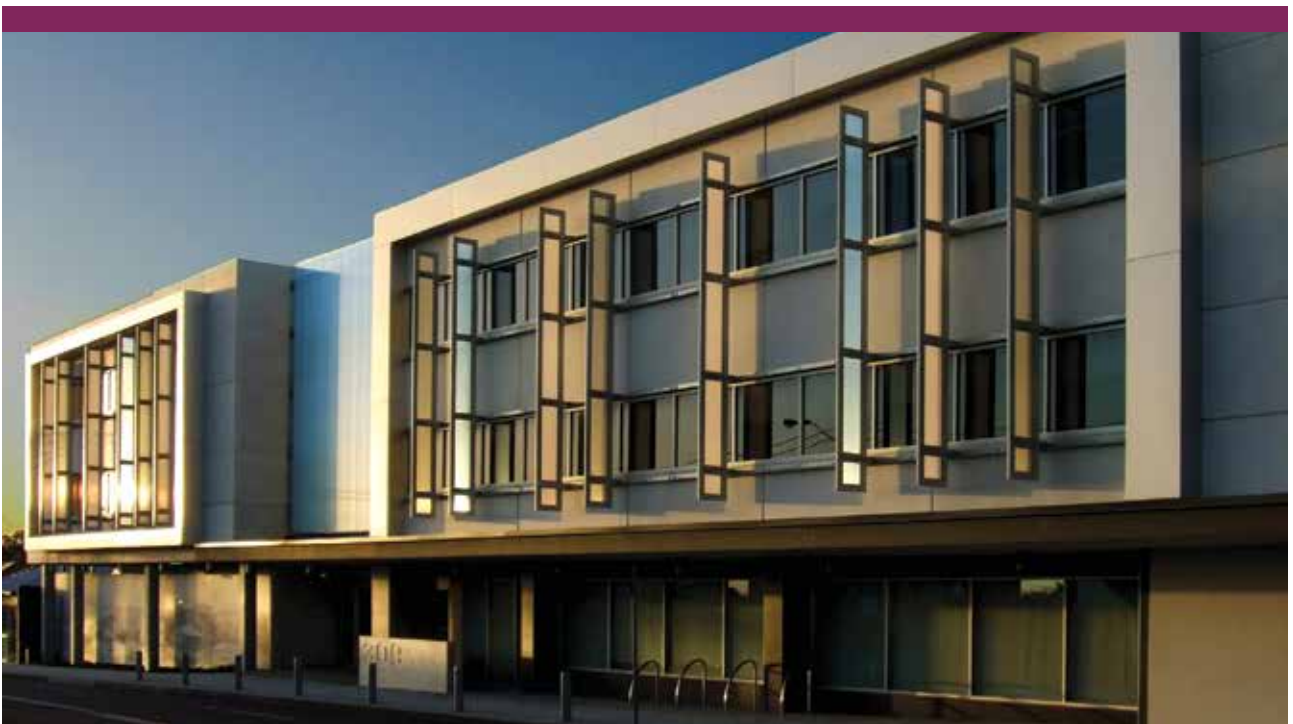
Community Services Offices, Charlestown Australia | Danpal® Louvre System | Architects: Jackson Teece
